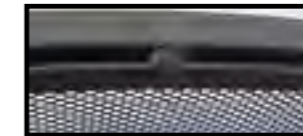
Mesh fitted between main frame and welded strip at rear
